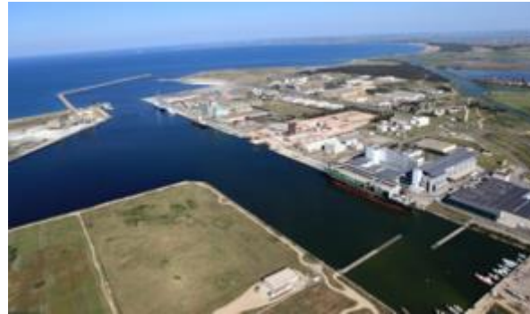
Industrial and manufacturing site
